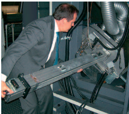
Thomas Unterberger, Chief Technical Officer, Herold Druck und Verlag AG, Vienna/Austria handling a lamp module of the Eltex INNOCURE Inert UV dryer installed on a press extension.
